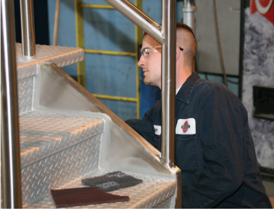
▲ Another large portion of Shickel Corp.'s business is fabricating components and installing them as well. These stairs are destined for a food processing plant.
